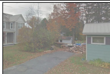
The small white building at the end of the driveway is the only remaining structure of the old Fairgrounds.
