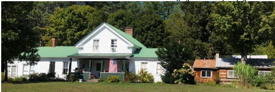
Stephen Griffing homestead today, front facing the river and wings added by Nathaniel Griffing in 1850. Log cabin close by.
