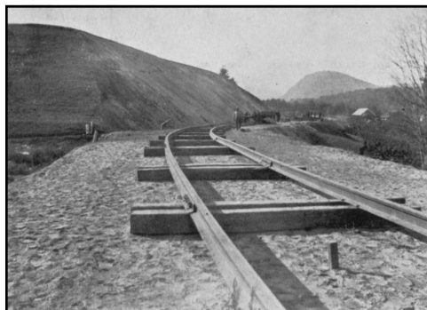
Newly laid track near Warrensburgh
