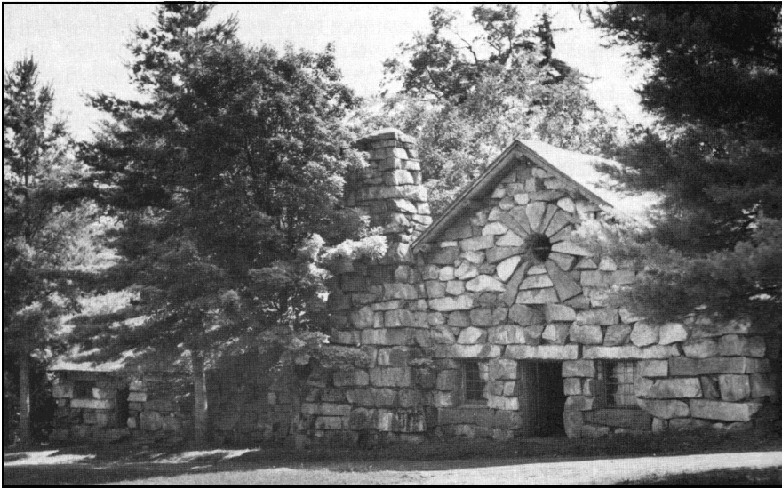
Cyclopedean construction, named for the large stone size, at Kamp Kill Kare from Durant
